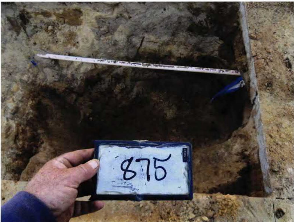
Picture 2: UST 875Cobia excavation.
